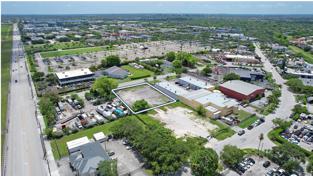
Subject outlined in blue. SW 143rd Court, between SW 141st and SW 142nd Streets.
