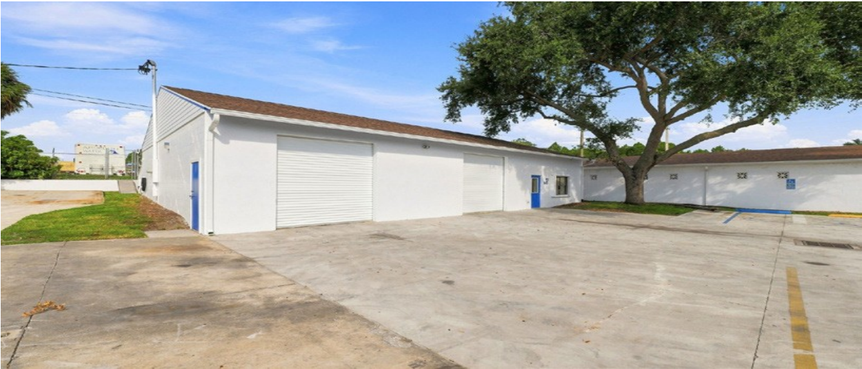
Freshly painted elevation with separate office entry
