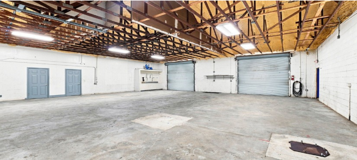
12-foot ceilings, two roll-up bays and drive-through access
