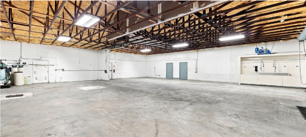
Full shop depth with direct doors into the office suite
