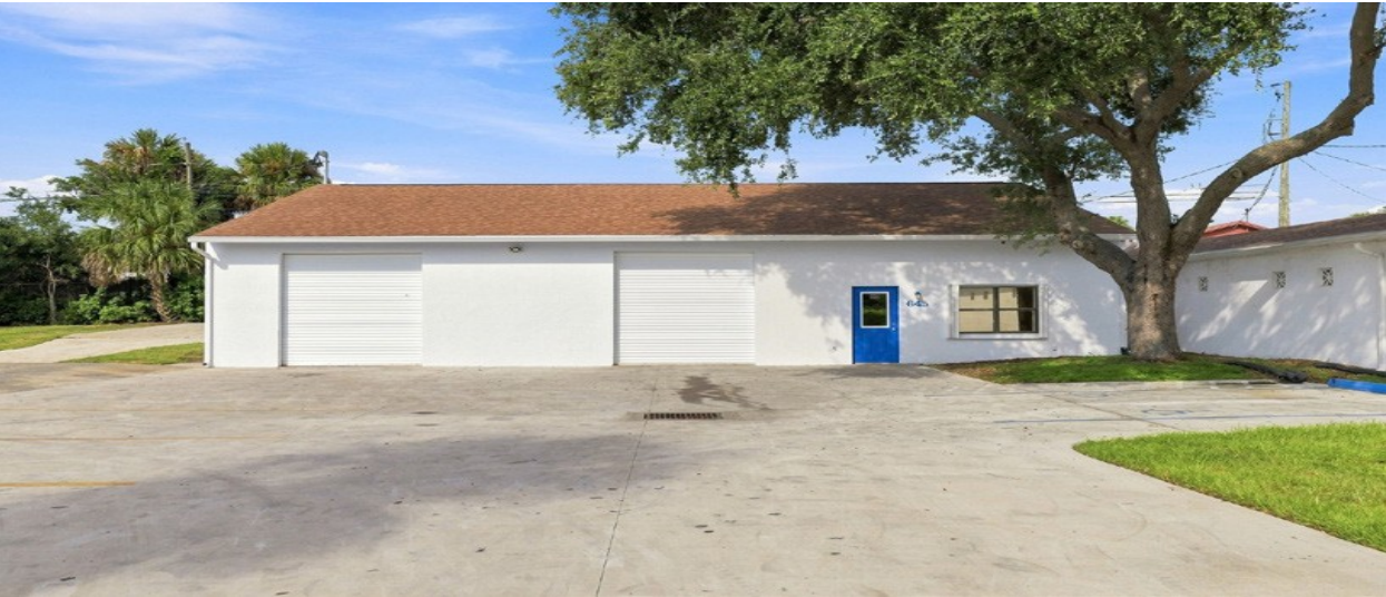
Full frontage: gated entry, concrete apron and two roll-up bays
