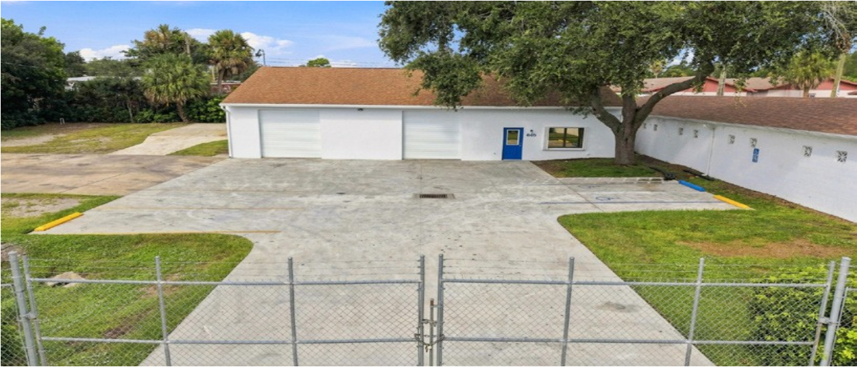
Security fencing and gate, well lit at night
