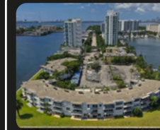
MACKLOWE DEVELOPMENT SITE
