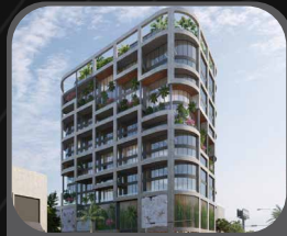
THE URSA 30 NE 39th St Class-A Office Space
