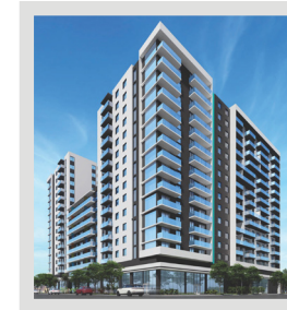
Urban 22 started Construction – 422 Multifamily Project
