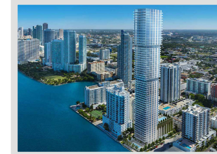
57 Story Elysee Tower Completed
