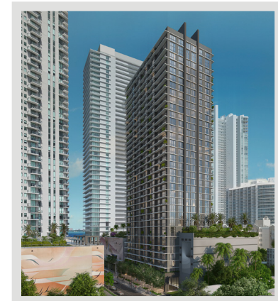
32 Story Metro Edgewater Begins Construction
